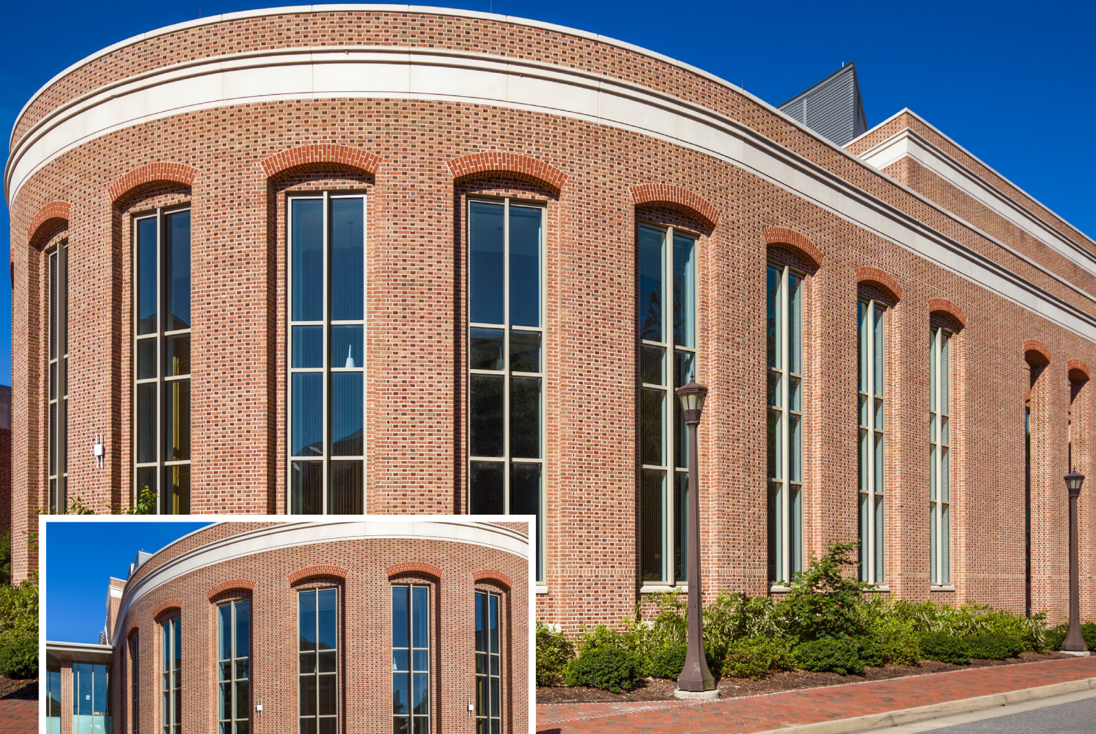
Santa Fe Mods (field brick), Hunt Valley (headers in flemish bond pattern) and Camden Blend arches.
