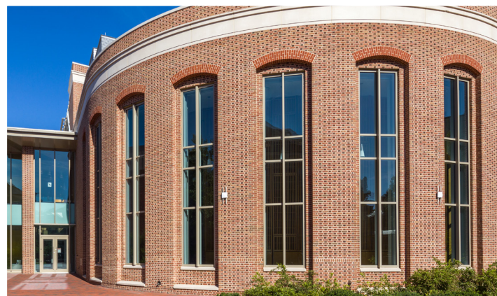
Santa Fe Mods (field brick), Hunt Valley (headers in flemish bond pattern) and Camden Blend arches.
