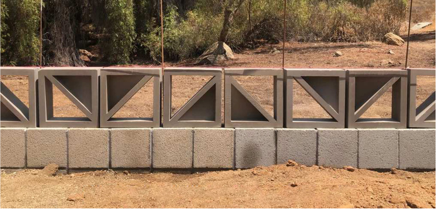
Blocks laid to check alignment
