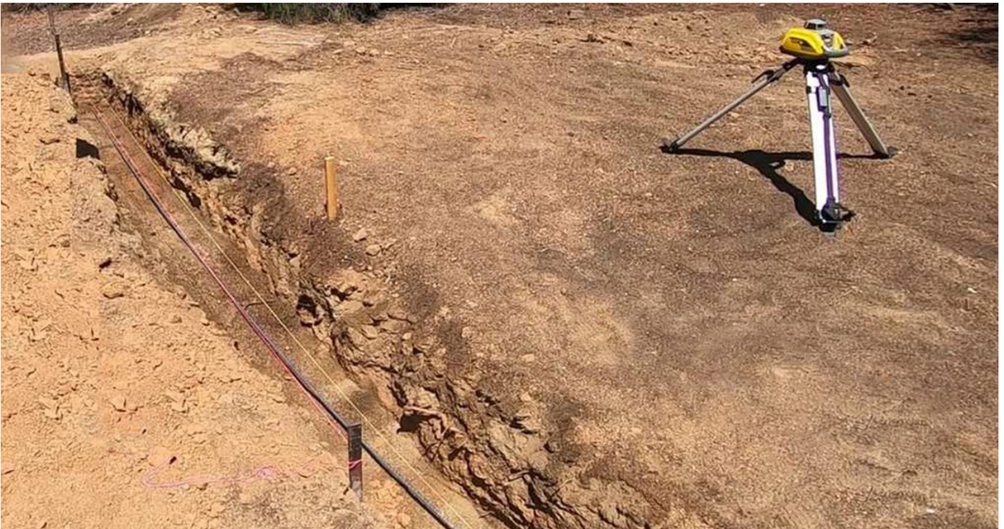
The trench for the footing
